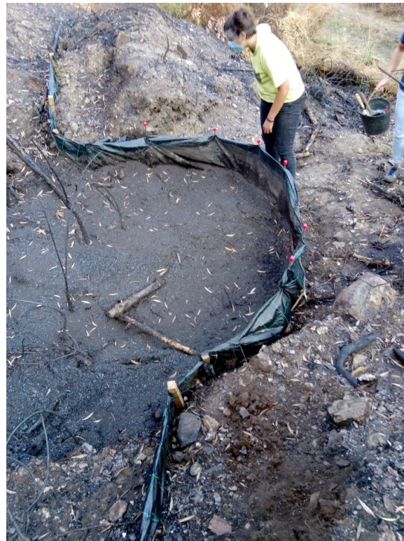
115 kg of eroded sediments captured by the sediment fence at the outlet of one of the EPyRIS swales in the Penouços burnt area - these sediments were produced by the first post-fire rainfall event and are black because they contain much wildfire ash and charcoal
